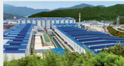
The Arvedi ESP process, produces hot strip in a combined, continuous, and uninterrupted casting and rolling process.
