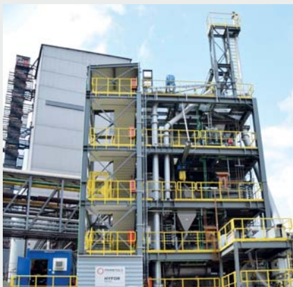
HYFOR is the world’s first direct reduction method for iron ore fines, eliminating the need for agglomeration processes such as sintering or pelletizing.
